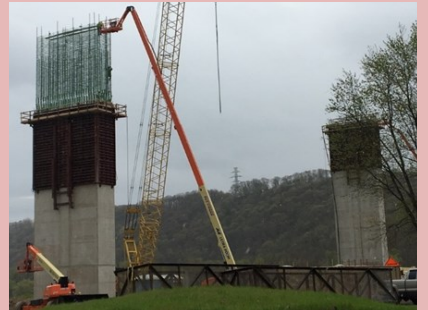
River Bridge Piers 4 and 5
